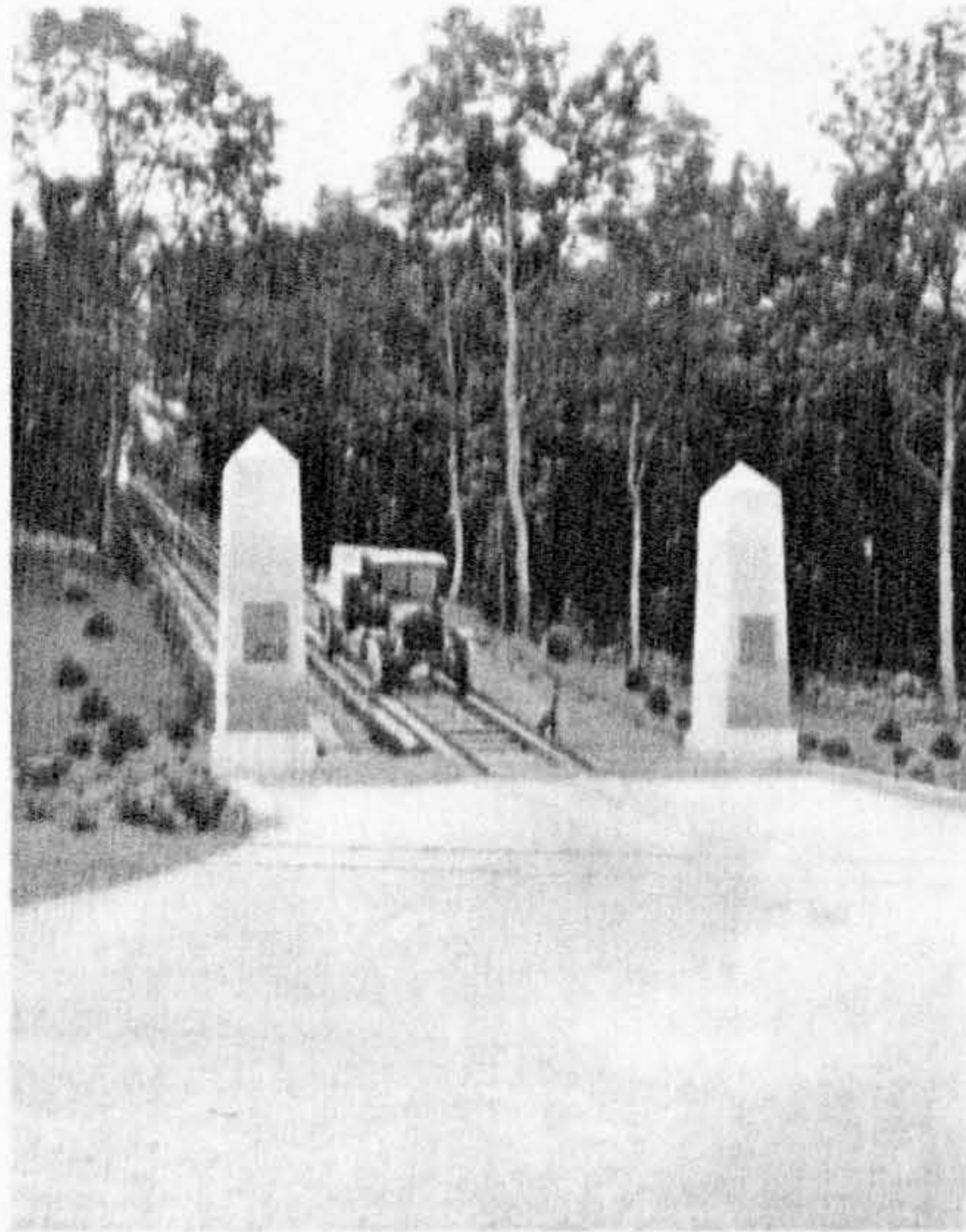
The Granite Rail Incline ca 1920
